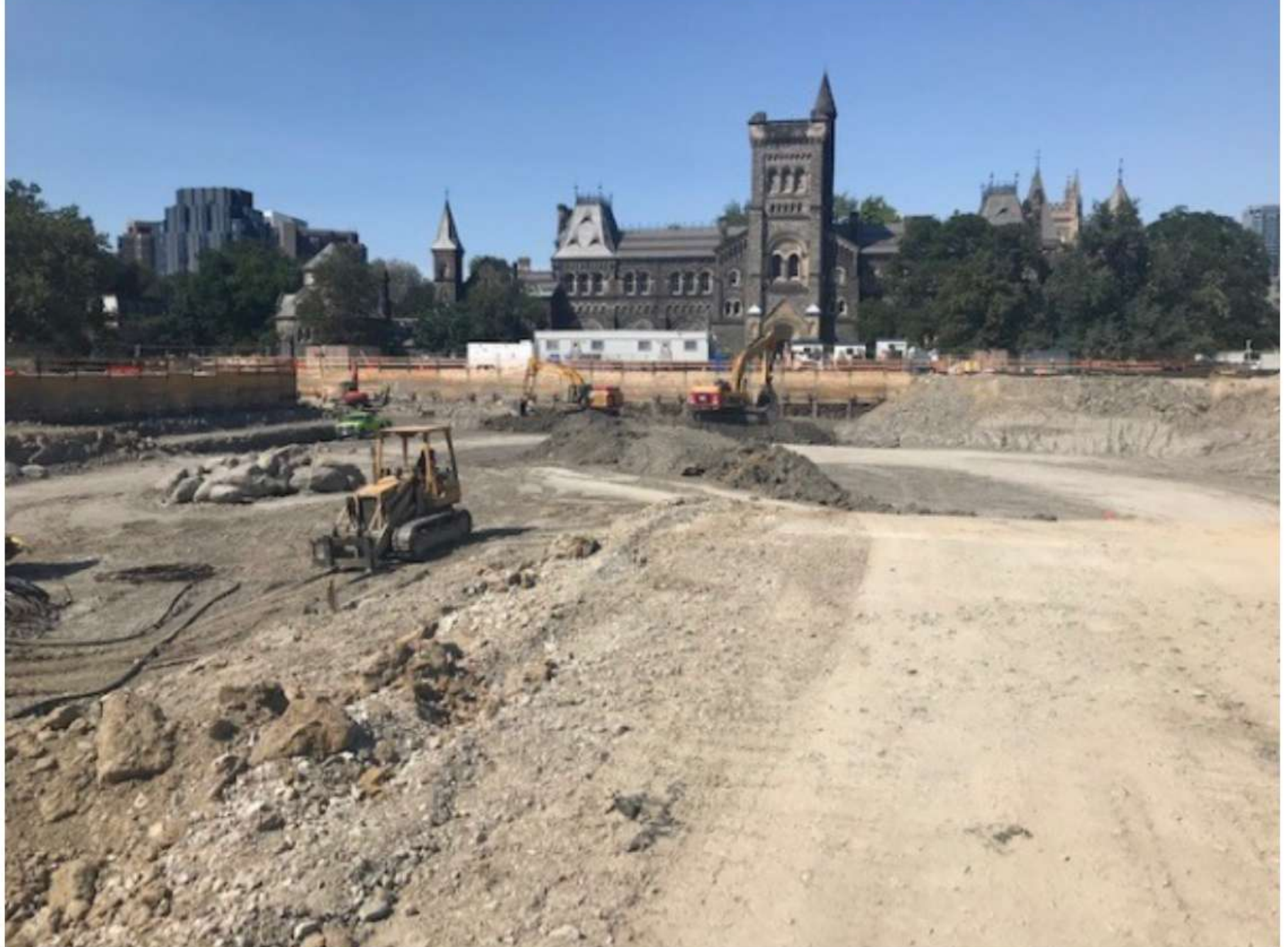
KCC excavation - September 2021
